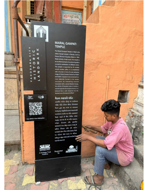
Installation of Signage at the Mairal Ganapati Temple
